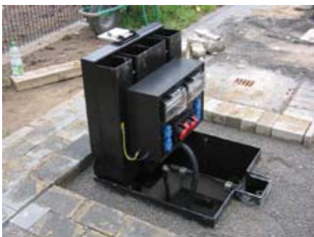
Filling up with gravel, concrete or other material
