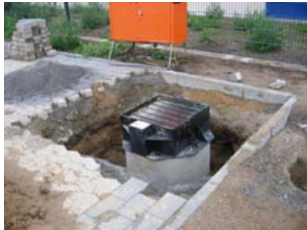
Insertion of the entire unit into the prepared hole
