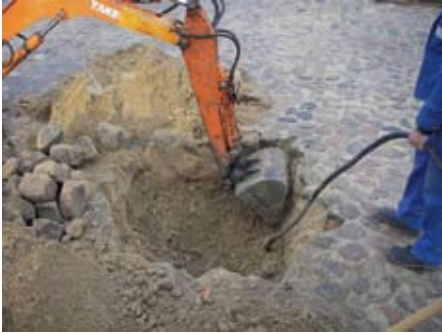
Excavation of the hole
