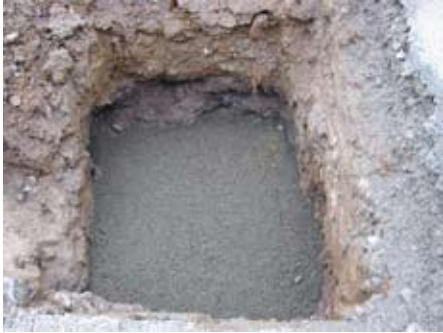
Excavation of the hole
